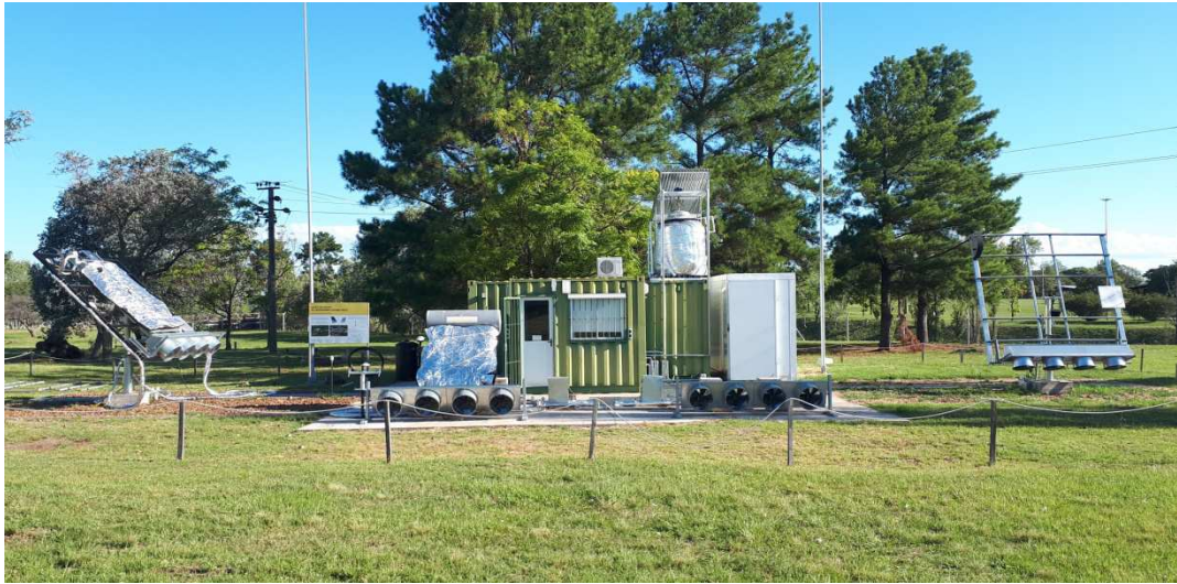
Fig. 1: Solar Water Heaters test facility installed in Uruguay.
